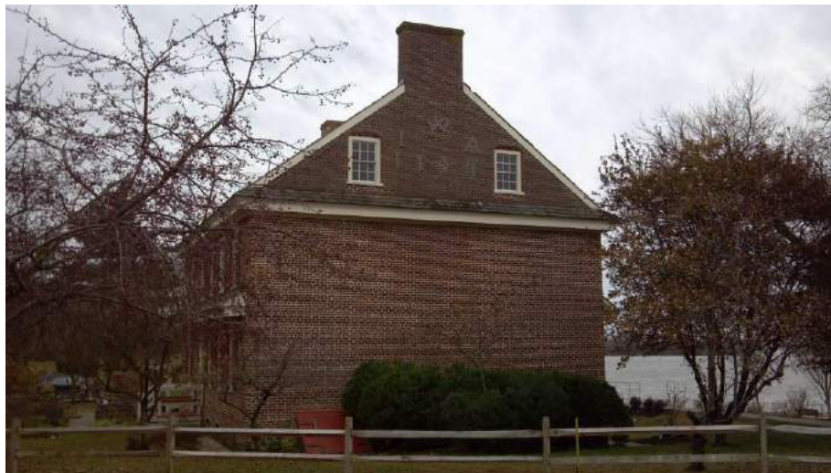
Figure 35. James Whitall House, north elevation, Delaware River in background.
