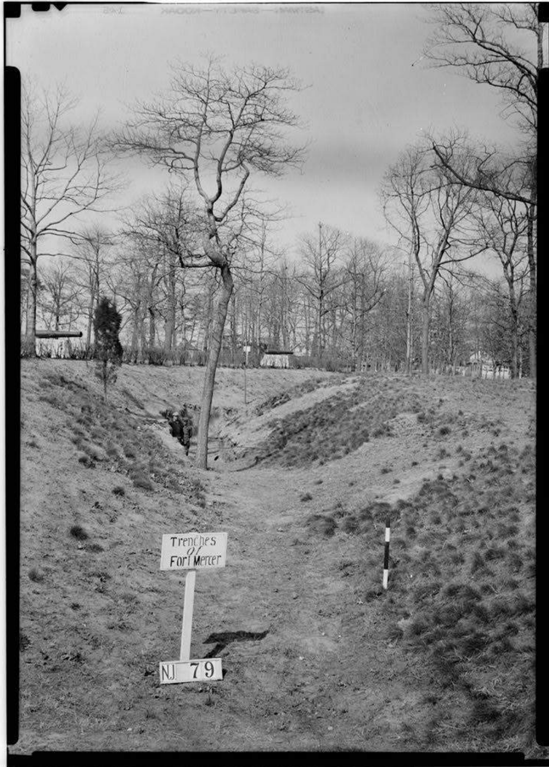
Figure 86. Photograph from the Historic American Building Survey documentation, showing workmen excavating in the Fort Mercer trench (HABS 1935).
