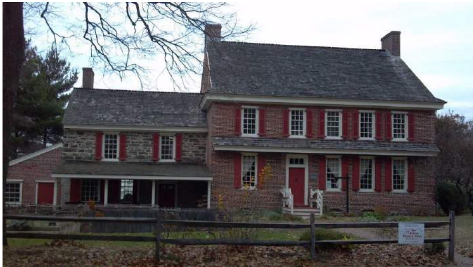
Figure 34. James Whitall House, east elevation, from Hessian Avenue.
